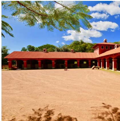
14 Stalls + Tack Room
